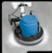
Smoothing and restoration of concrete screed
